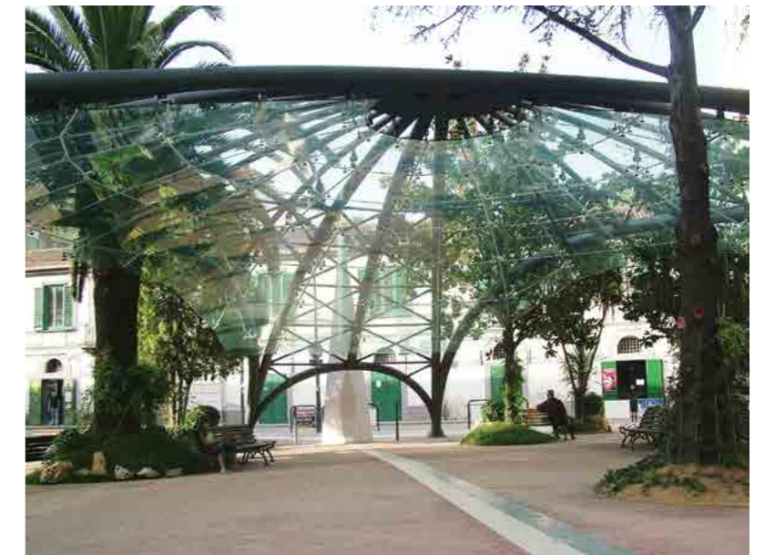
Covered square in Pontecagnano (SA). Place couverte à Pontecagnano (SA).
